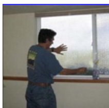
Smooth bubble wrap out so that water contact holds it in place.
